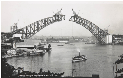
Figure: Sydney Harbour Bridge under construction [NMA]
