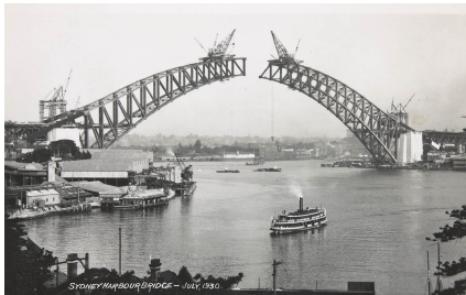
Figure: Sydney Harbour Bridge under construction [NMA]
